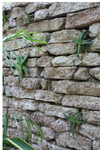
Aloe saponaria planted during construction
