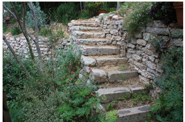
Steps from salvaged saw-cut curb pieces will be faced with flagstone veneer
