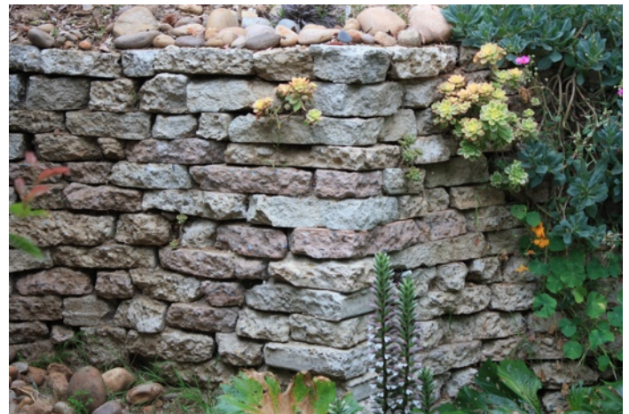
Completed wall incorporating colored concrete pieces
