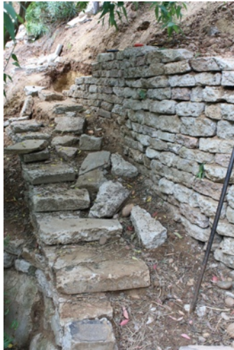
Step and wall construction
