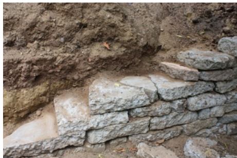
Overlapping pieces of concrete
