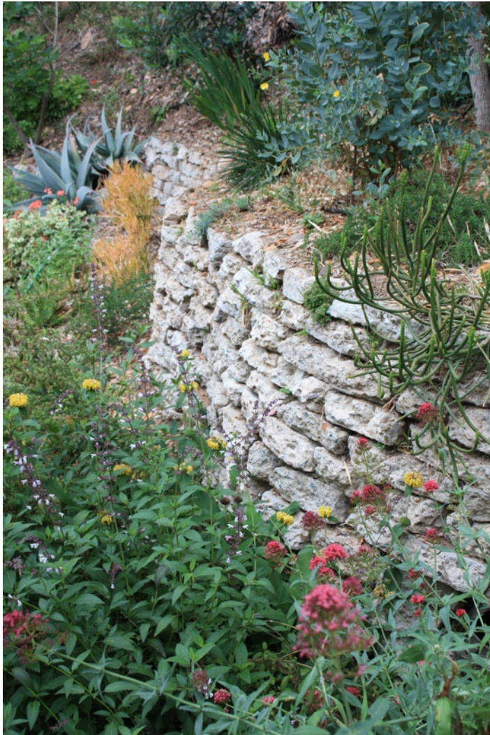
Completed wall with sloping grade above
